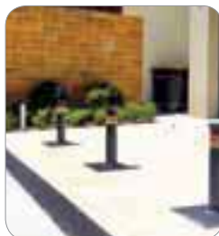
Instalace sloupu Coral
